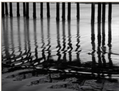
PIER PILINGS 14 PSPSN-141
